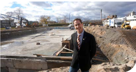
We're renovating the Parkhaven Pool this fall and winter.
