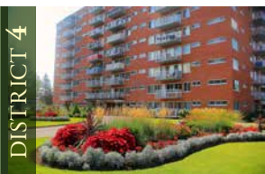
DISTRICT 4 Highrise Building 7461 Kingsley
