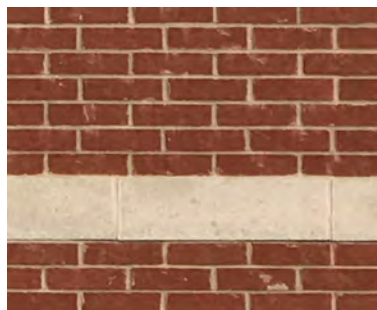
Stone ledge/band on a masonry wall
